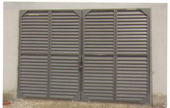
Substation Main Entrance Gate - 4m (W) x 3m (H)
